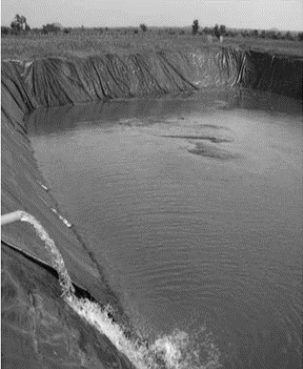
Construction of pond for irrigation
